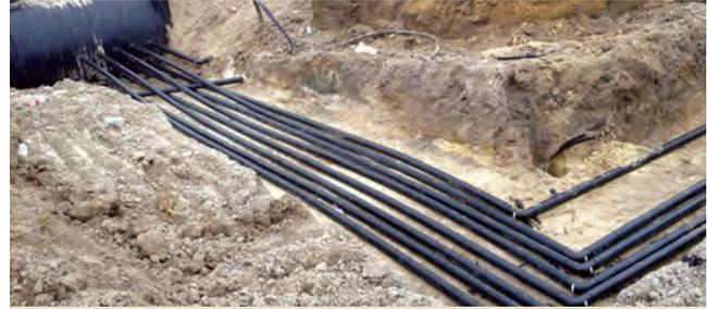
**PHOTO 1** Horizontal HDPE piping, trenched at minimum 4 ft (1.2 m) below the grade level, connects the supply and return piping from each bore hole to the HDPE vault in a reverse-return arrangement, which minimizes system pressure drop and the corresponding pumping energy.
